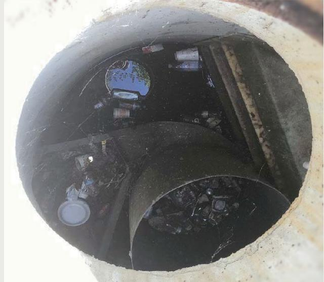
Technicians carefully open, monitor, and treat an underground BMP. A close picture shows how trash and other contaminants can pile up in these devices.
